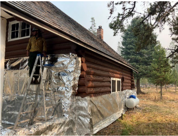
Stolle Meadows structure Getting Wrapped for Fire
