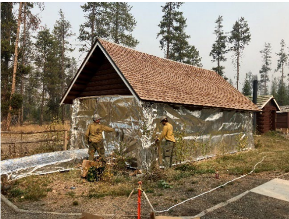
Stolle Meadows Getting Wrapped for Fire Suppression
